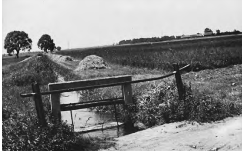
View from the wide bridge (‘Weidbrücke’) to the Hartenau farmstead. In the foreground is the weir at the creek (‘die Bach’ or ‘Landbach’). It served to irrigate the adjacent meadows in dry years. To the right of the creek the huge reed bed, now no longer there apart from a few hundred square metres. This view was likely c.1949.
