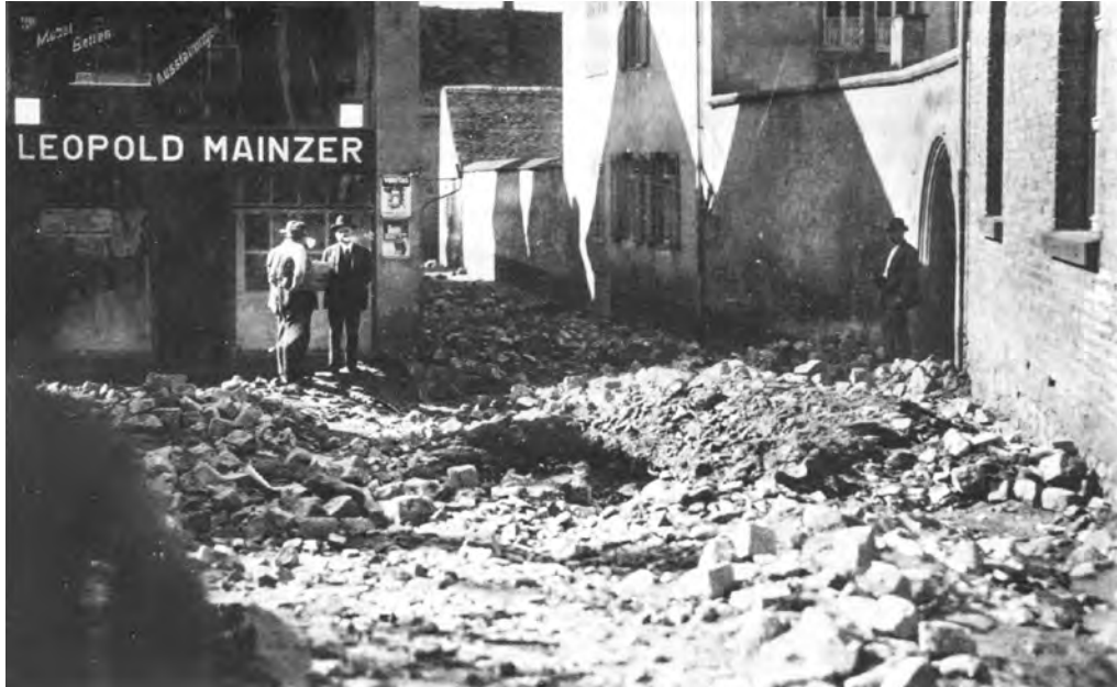
Storm damage in 1928 in Zwingenberg, corner of Obergasse and Untergasse.
